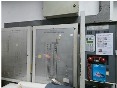
Fire Alarm Control Panel
